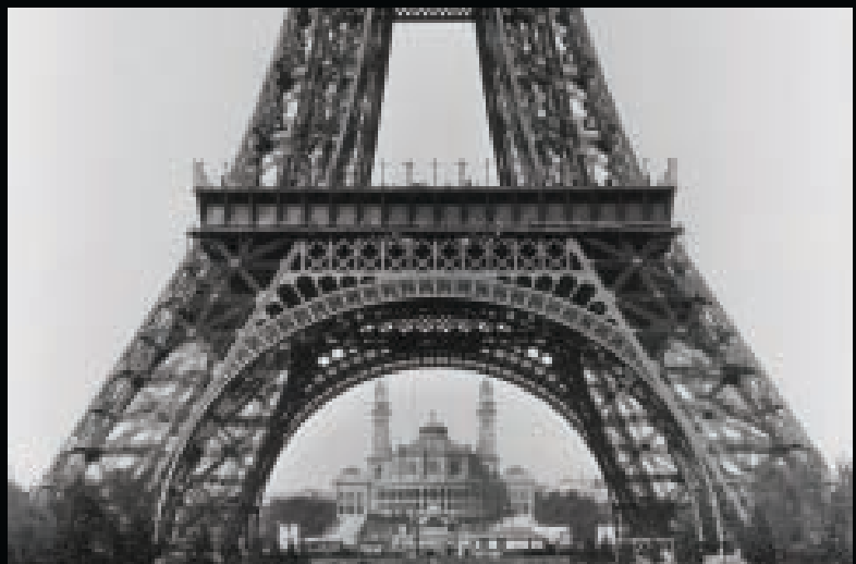
Two of Jean Dunand's influences. Above: the Eiffel Tower during construction. Image courtesy of Collection tour Eiffel. Top: Crystal Palace, home to the 1851 Great Exhibition.
